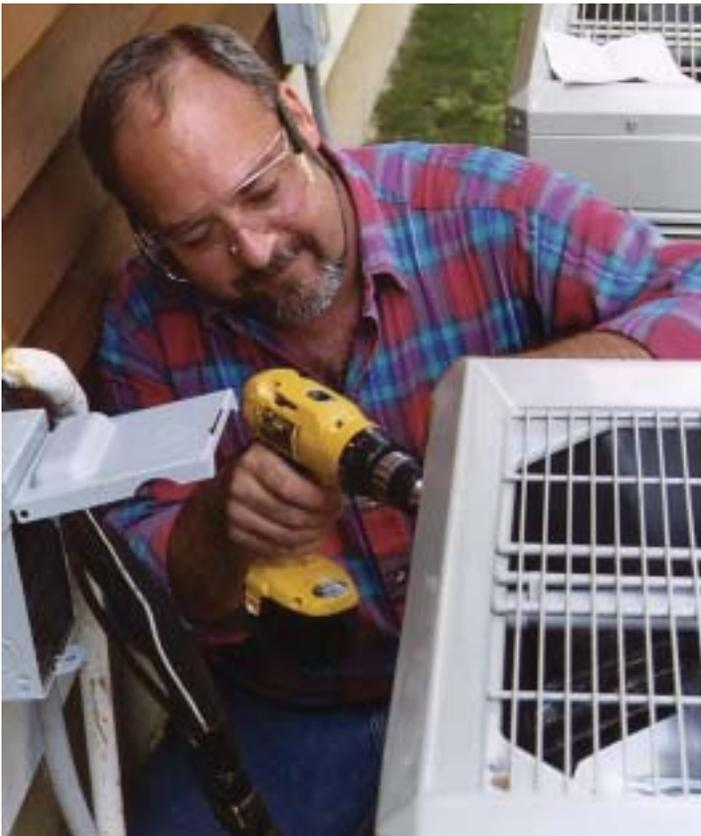
Top: Ron Eastwood of Eastwood Electric prepares the condenser for the installation of a head pressure controller. Safety first: switch off the disconnect. Above: Some models need to have the fan removed to access the coil and the wiring.
